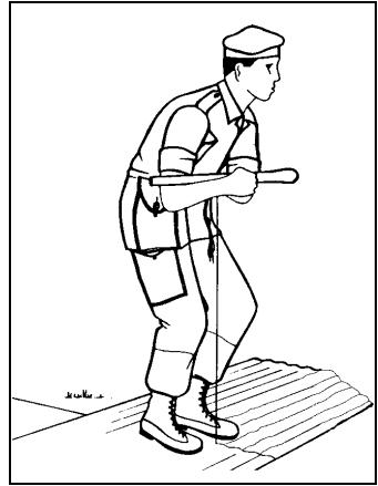
Fig 6-3-4 Cutting Corrugated Iron
