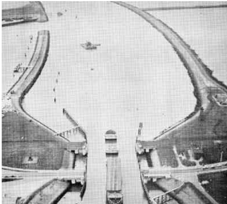
Figure 10-6 Low Angle Oblique Photograph
